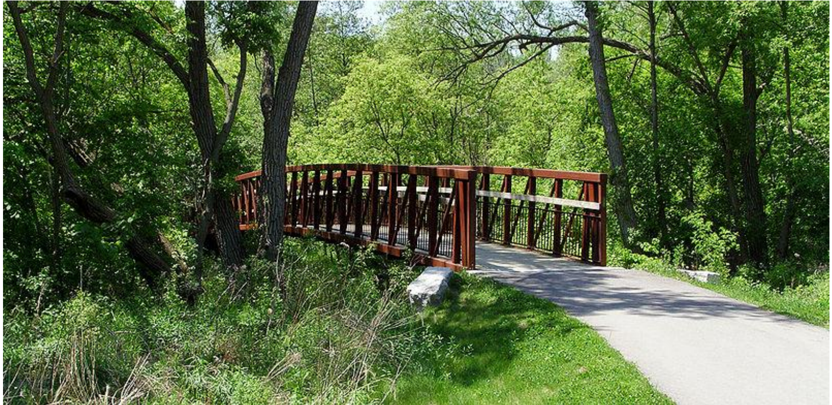
Engineered Steel Pedestrian Bridge Crossing
