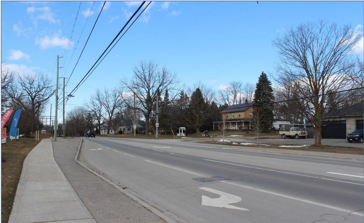
Photo 7: View northeast showing Leslie Street to the north of Manor Hampton Street and Colonel Wayling Boulevard
