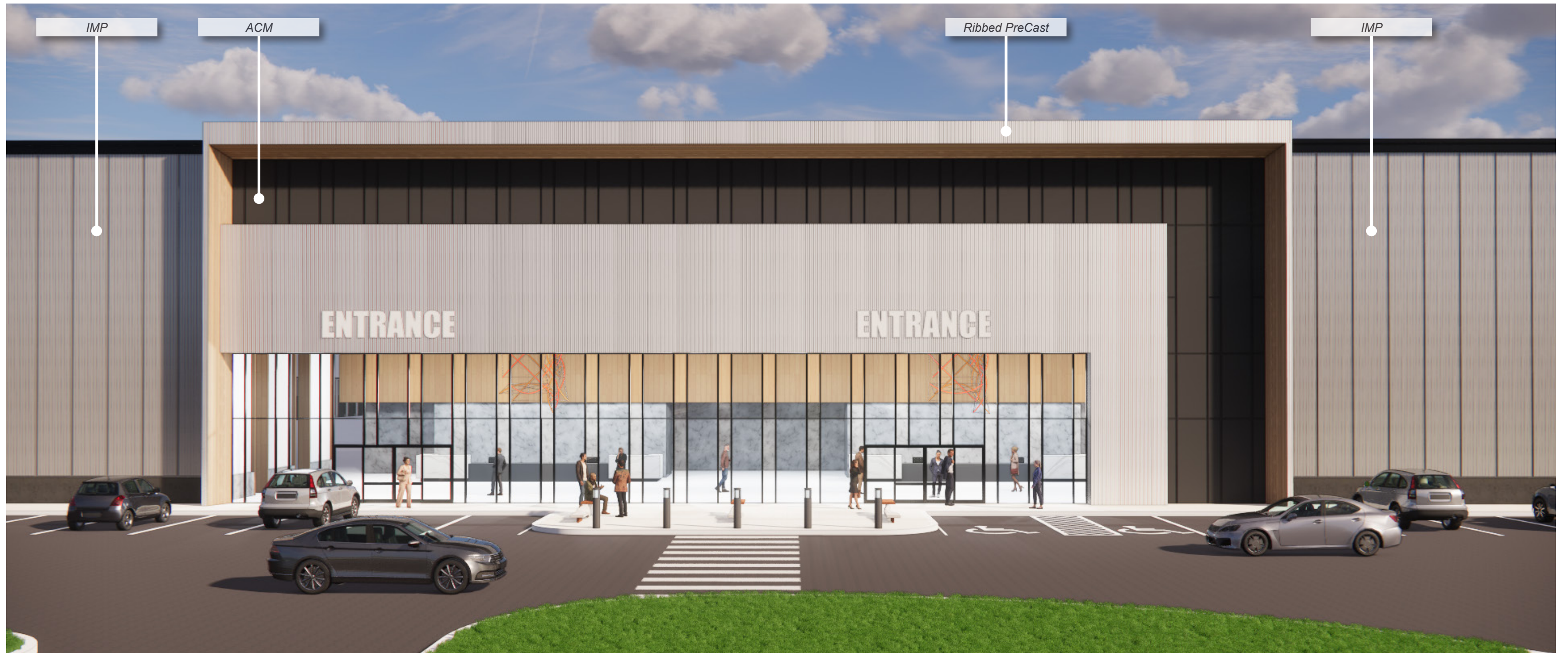
Office x Warehouse Entrance
