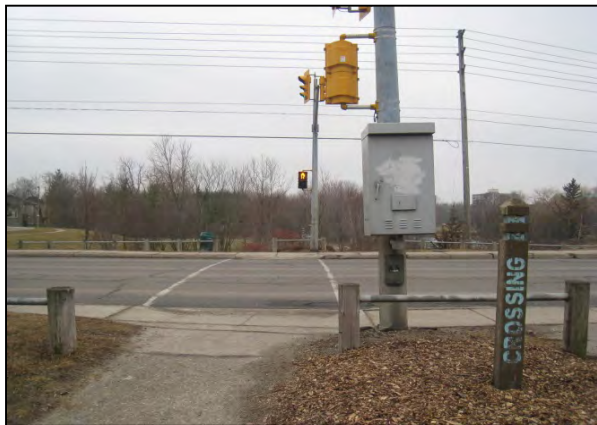
Photo Credit: MMM Group, 2012 – Mid-Block Pedestrian Signal without Median Refuge
