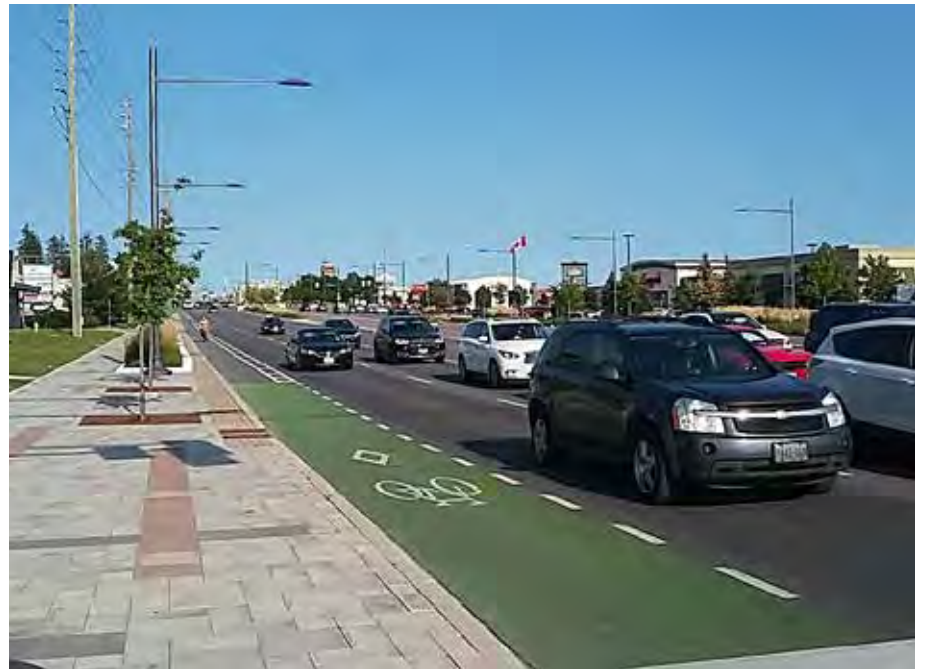
Highway 7 Bicycle Lanes
