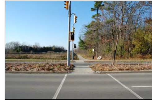
Photo Credit: MMM Group, 2010 – Mid-Block Pedestrian Signal with Median Refuge
