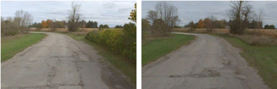
Figure A2 Pavement Condition
