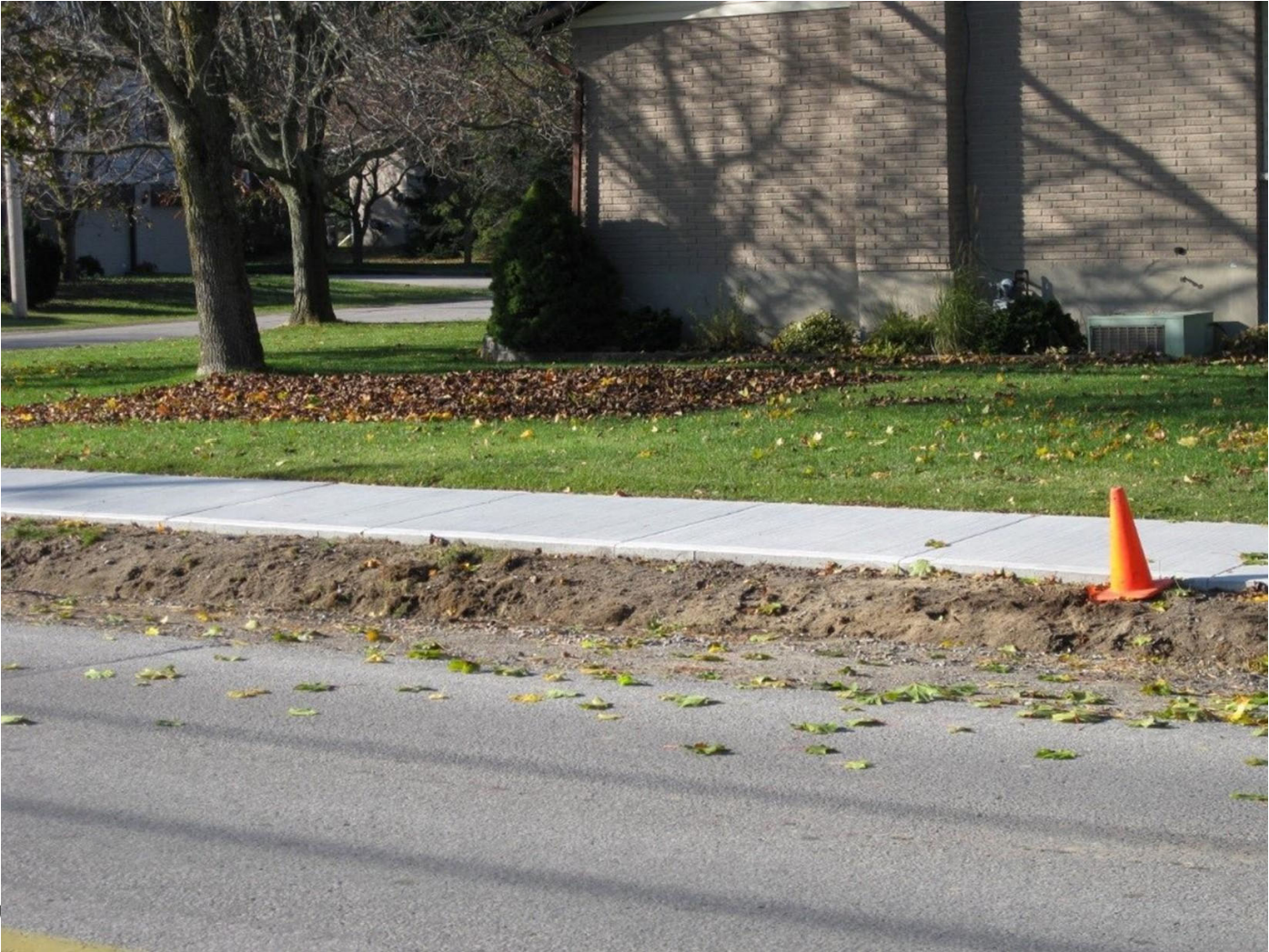
New Sidewalk Construction
