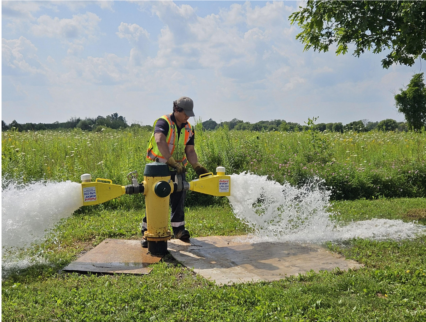
Hydrant Flushing
