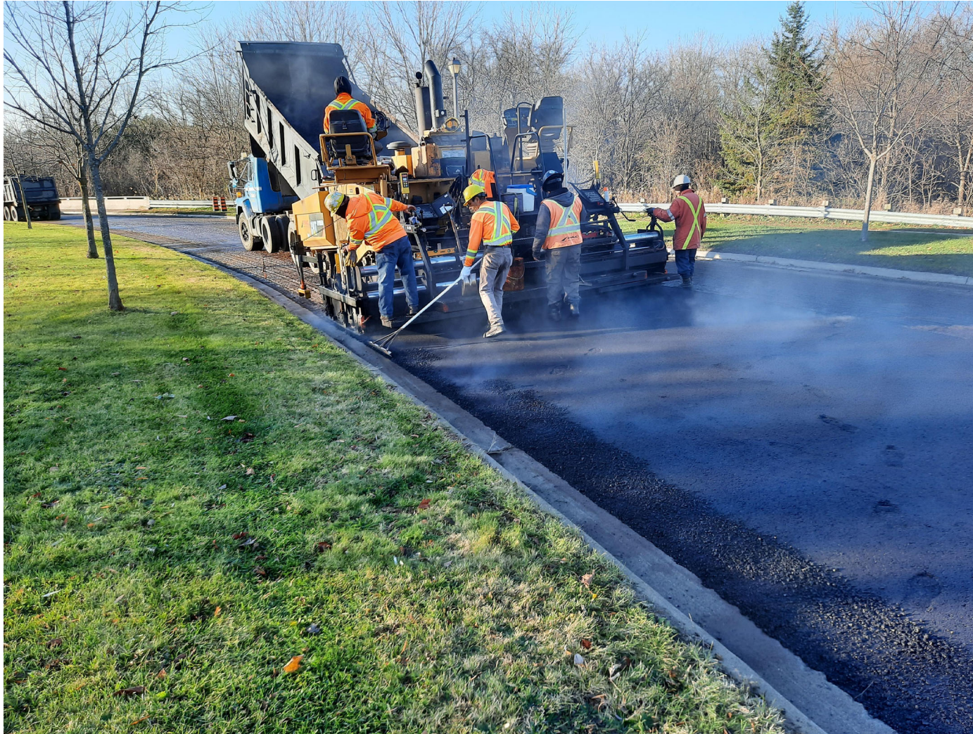
Asphalt Resurfacing 2
