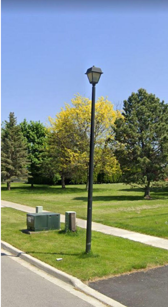
Steel Streetlight Pole
