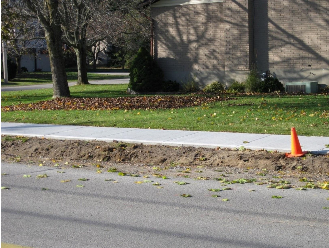
New Sidewalk Construction
