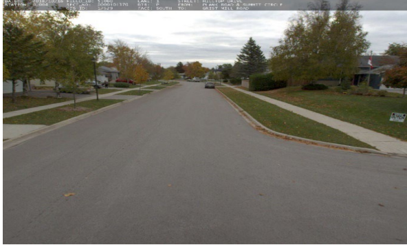
Figure 32: Images of Pavement Condition
