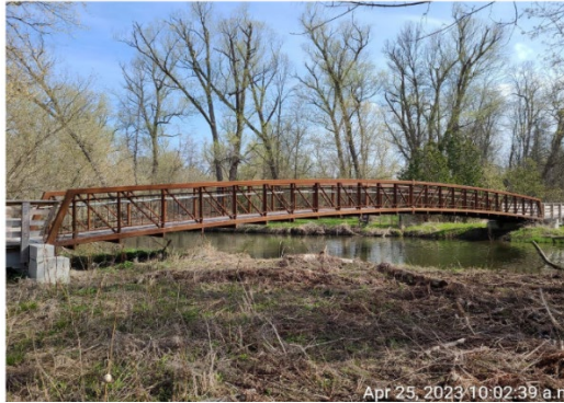
Figure 38: Images of Bridge and Culvert Condition
