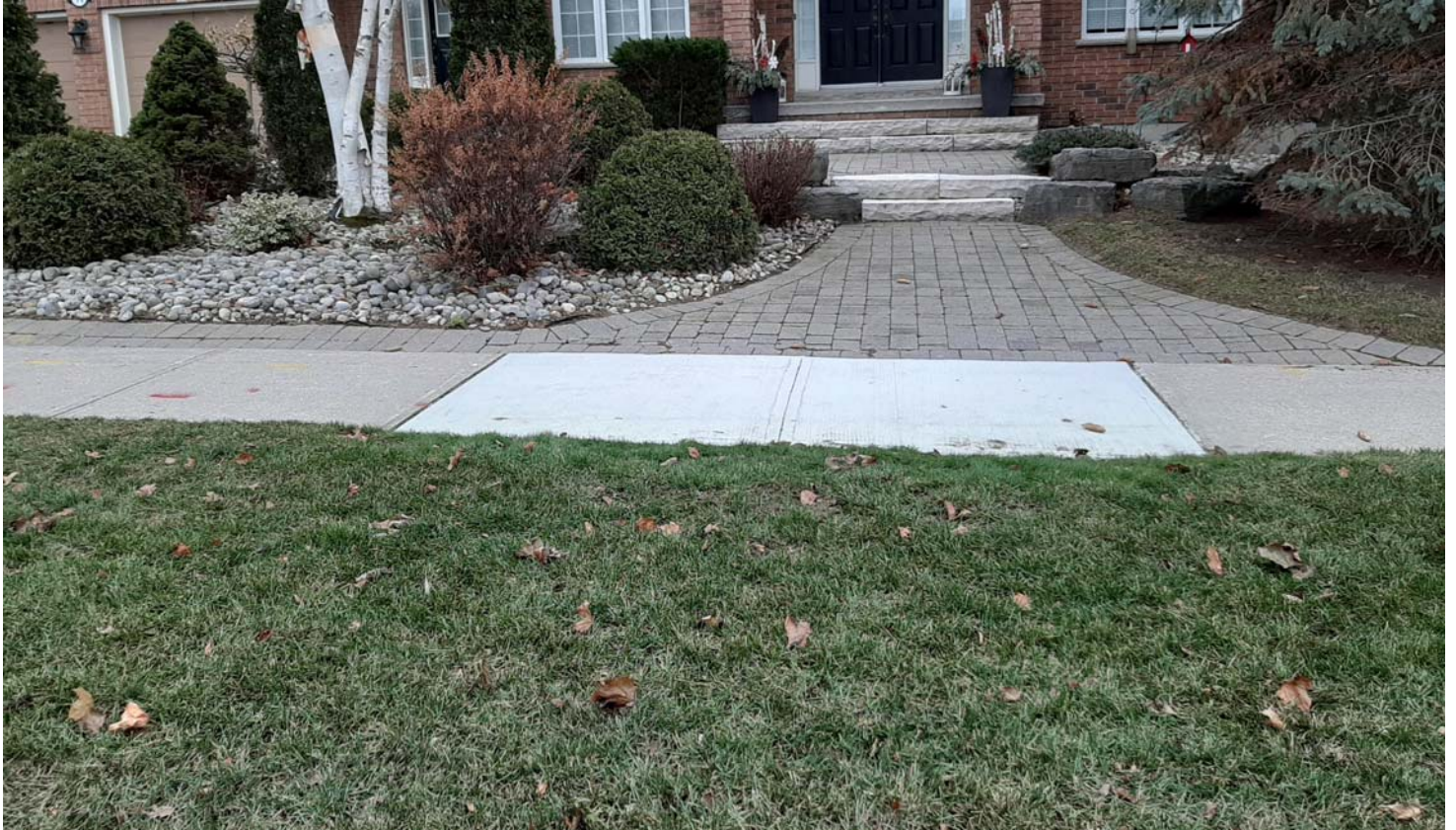
Misc. Concrete Rehabilitation 1
