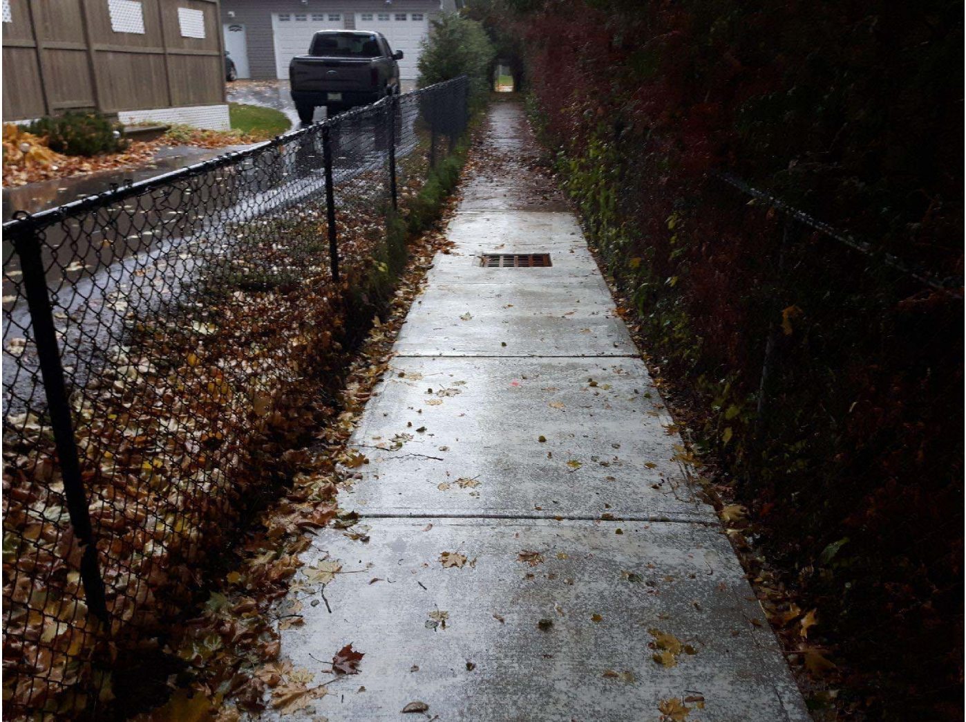
Misc. Concrete Rehabilitation 2
