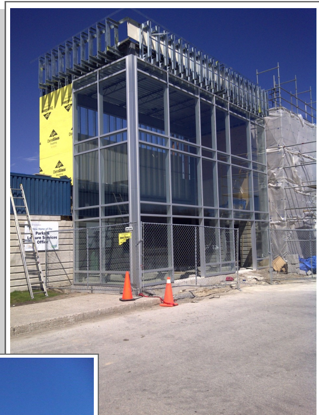
Glazing on the link and east entrance is complete.
