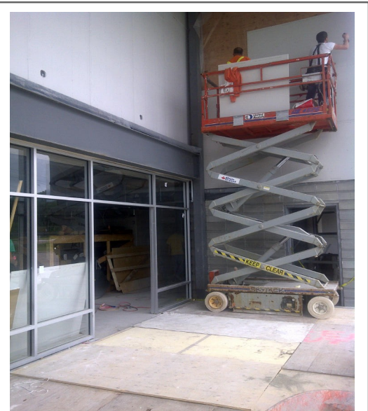
New Front Vestibule
