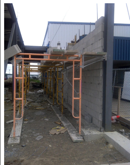
New West Community Hall being connected to West Arena
