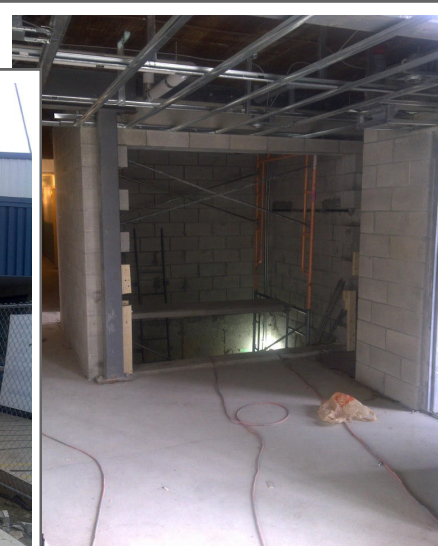
New Elevator Rough In
