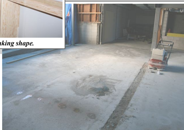
The main lobby subfloor being poured.
