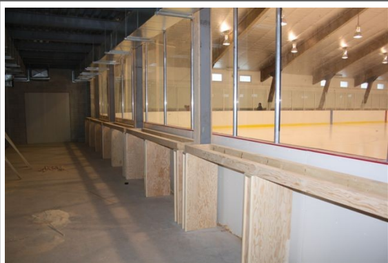
The east pad viewing area taking shape.
