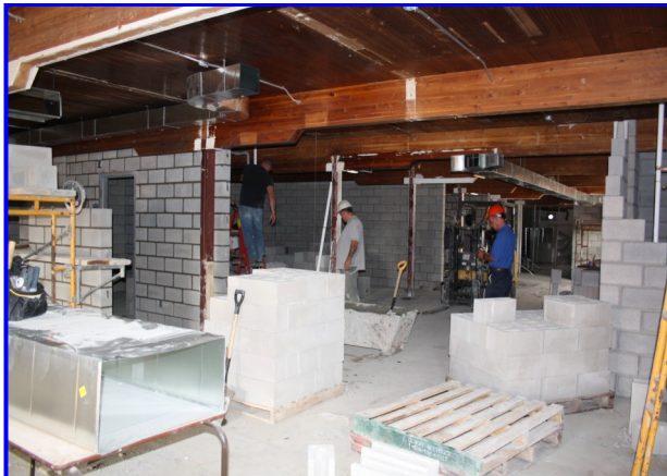
New dressing rooms being constructed
