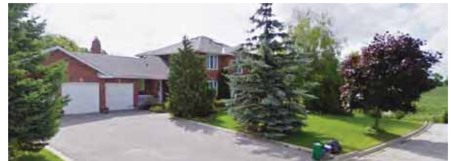
Civic Centre Drive
