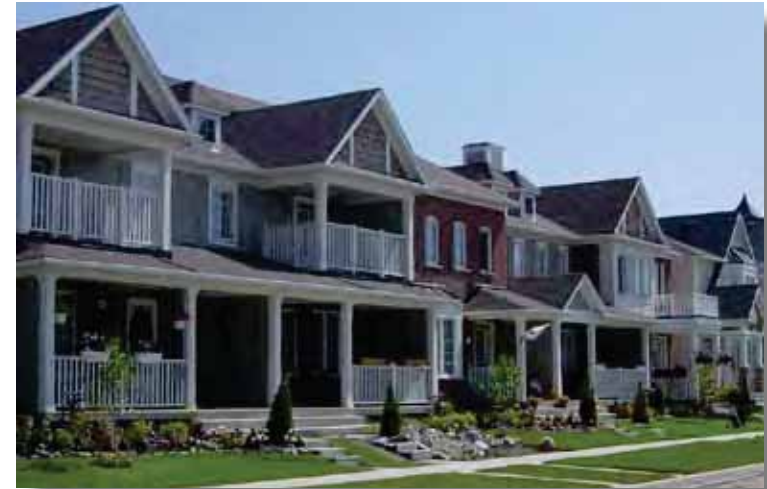
Dwellings with rear-accessed garages contribute to the streetscape appearance in key areas of the community
