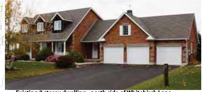
Existing 2 storey dwelling - north side of Whitebirch Lane.
