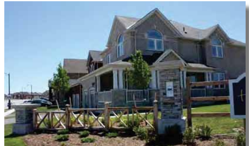
Gateway Dwellings shall be designed with high degree of articulation and detailing
