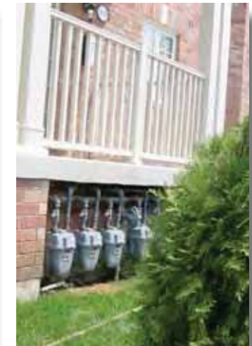
For Townhouses and other higher density forms, utility meters should be architecturally integrated or screened
