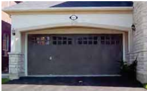
Image of 4.8m wide garage door patterned to appear as 2 single doors
