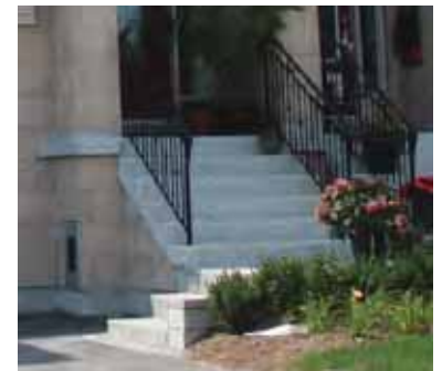
Poured-in-place stairs with masonry veneering on sides
