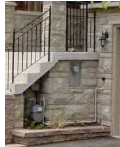
For Townhouses and other higher density forms, utility meters should be architecturally integrated or screened
