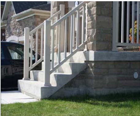
Figure 2.4d – Appearance of poured-in-place steps
