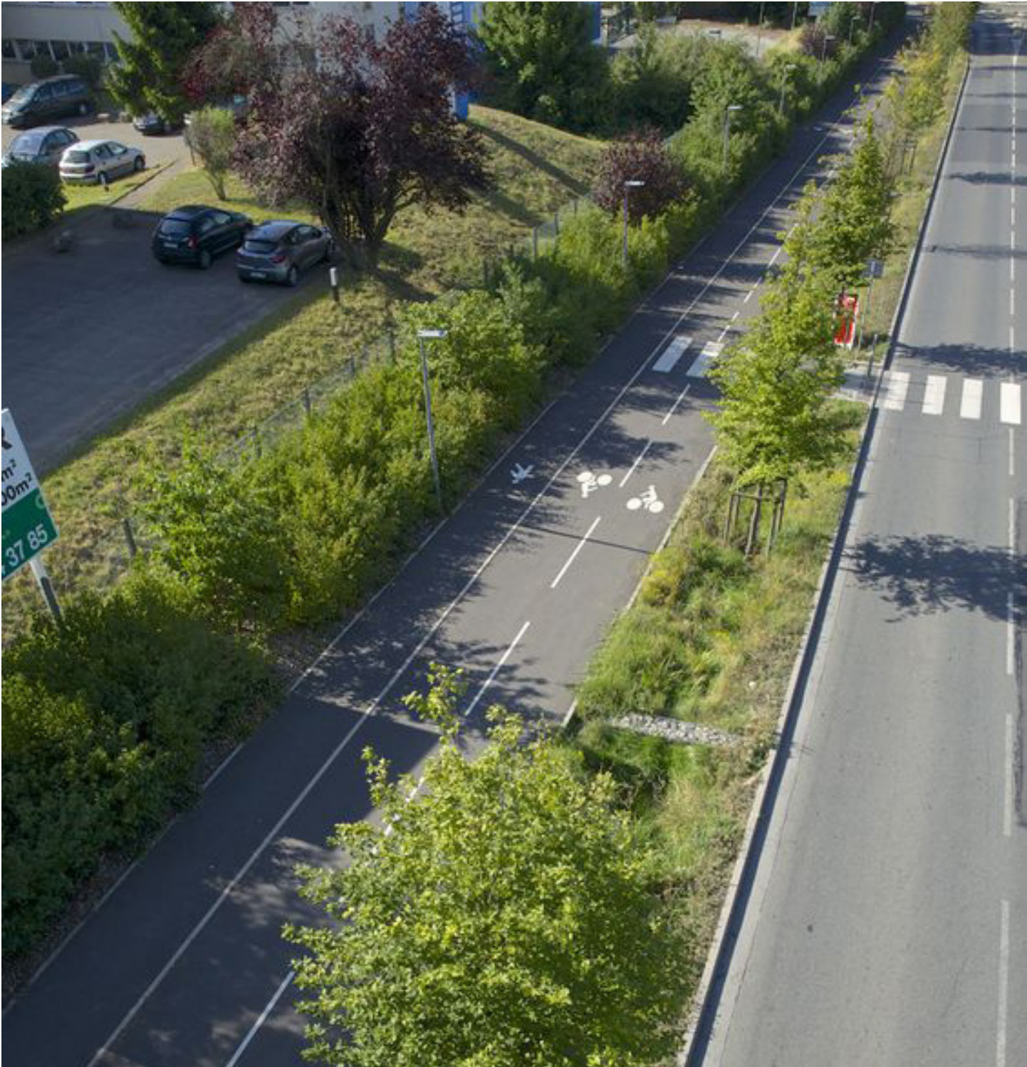
An example of a multi-use trail along a Collector Street
