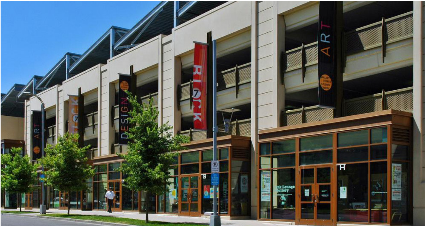
An example of building uses wrapping the facade of a parking structure
