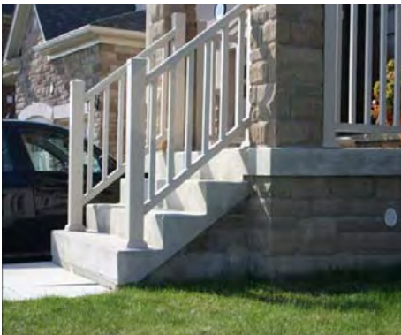
Figure 2.4d – Appearance of poured-in-place steps
