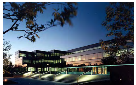
Figure 5.7 – Example of Lighting
