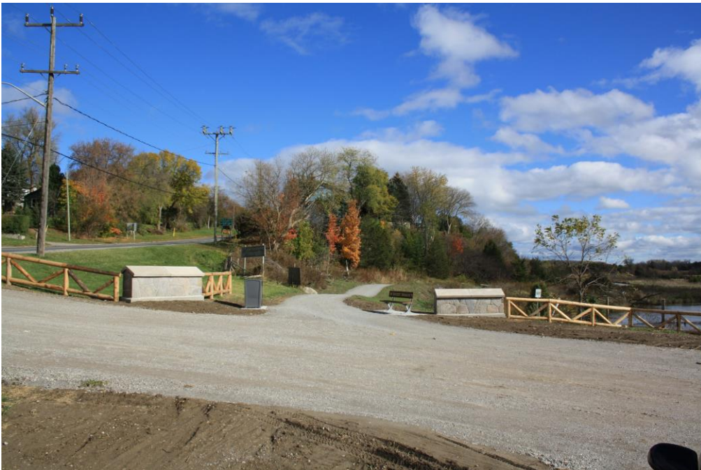
Trail Head and Parking Lot at Nokiidaa Trail – East Gwillimbury Partnership project with York Region. Promoting Active Transportation and Recreation
