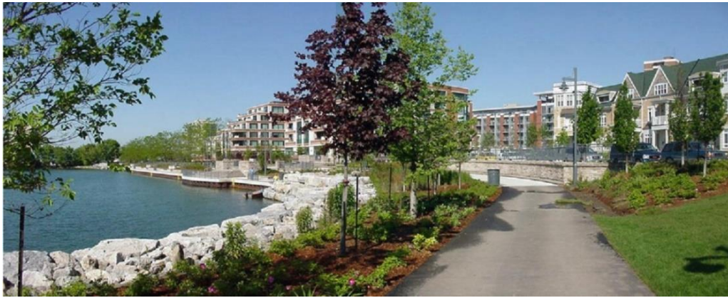
Waterfront pathways with erosion protection, landscaping and many seating options utilize natural features and enhances user experience.
