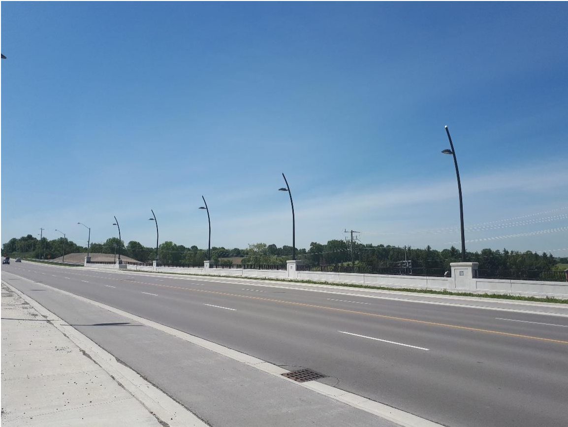
On Street Raised Curb Cycle Tracks at 2 nd Concession – East Gwillimbury Promoting Active Transportation and Recreation. Partnership Project with York Region
