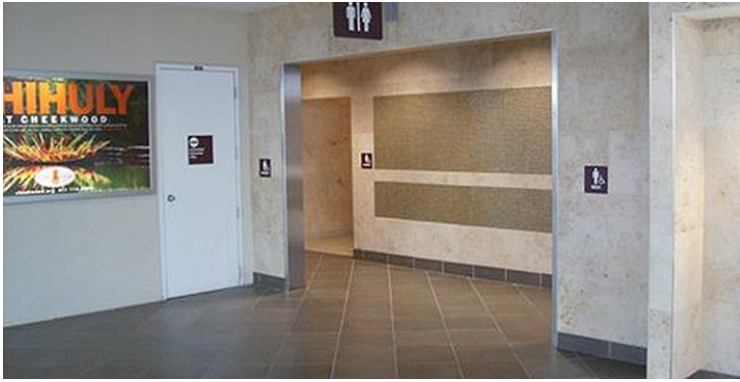
Example of a barrier free entrance.
