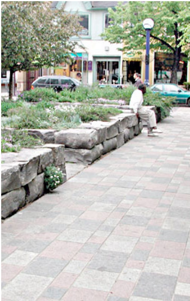
Light coloured pavers assist with the reduction of the heat island effect.
