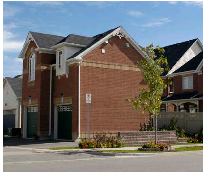
Detached garage with second storey dwelling unit.
