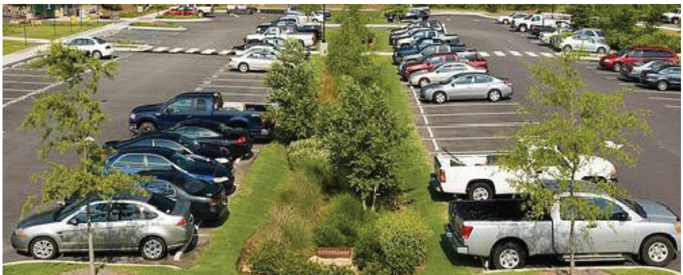
Example of a parking lot that incorporates planting strips for as a stormwater management strategy.
