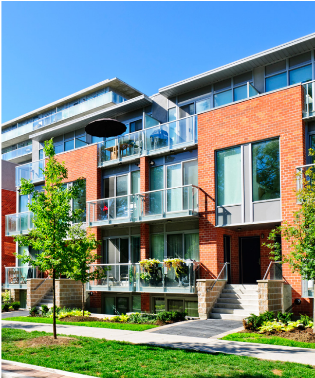
Stacked townhouses with balconies and entrances along the street.
