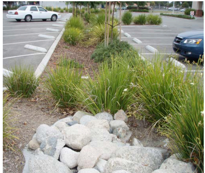
Landscaped island with a bioswale to filter run-off from the parking lot.
