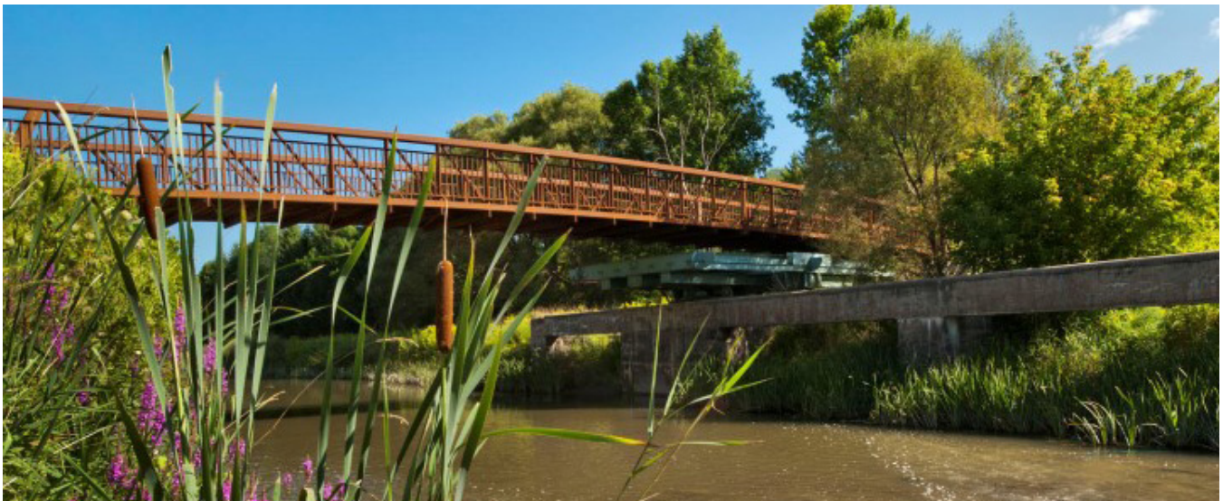
Nokiidaa Trail bridge.
