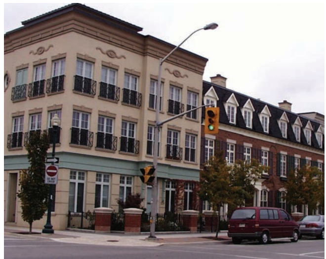
A consistent building setback frames the street..
