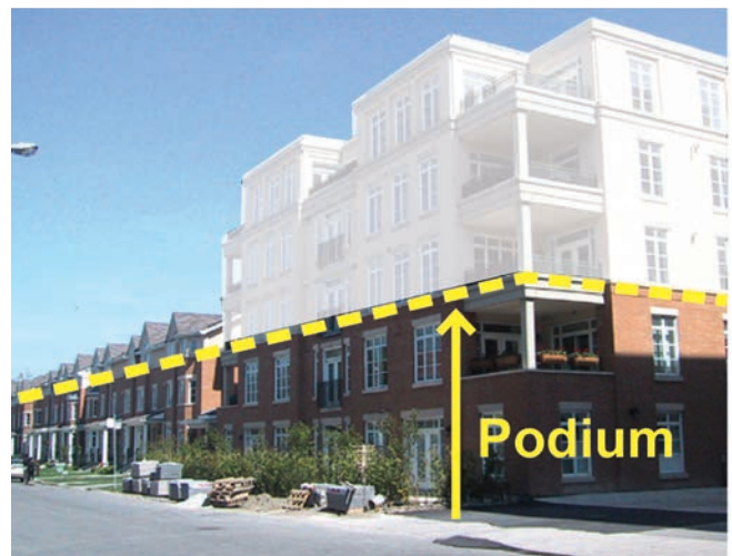
The height of the podium on the mid-rise building should match the adjacent dwellings.
