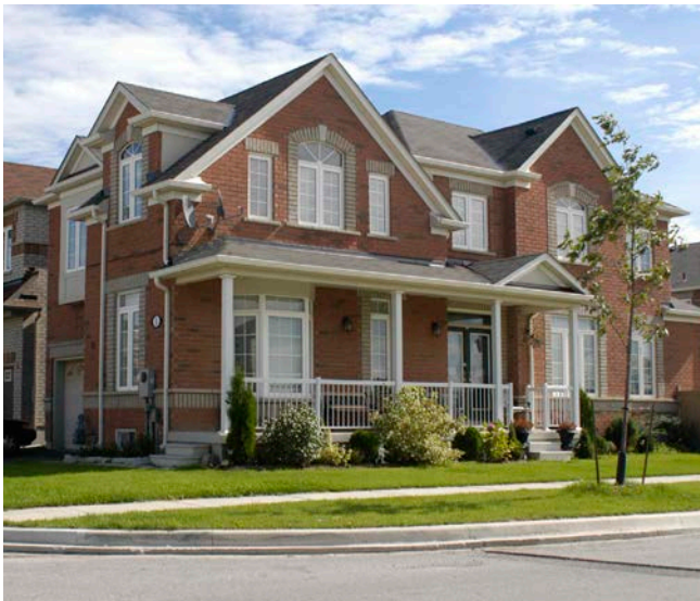
Single detached dwelling with upgraded side elevation.
