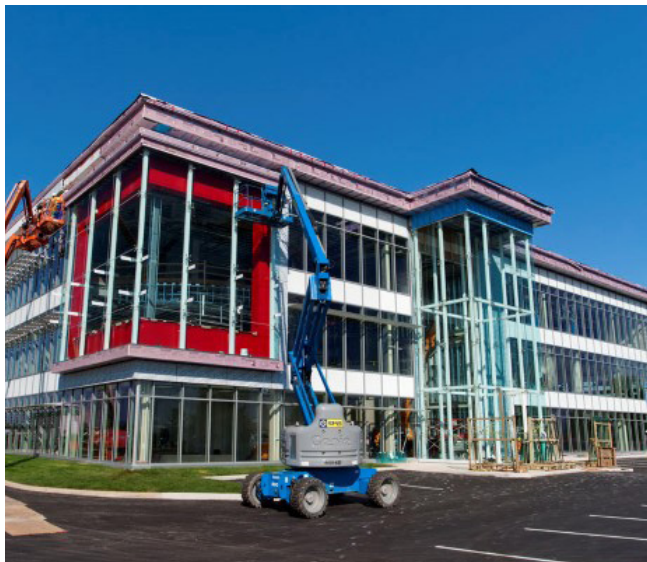
Construction of an employment office building.
