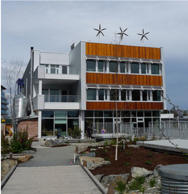
Wind turbines on the roof of an office building.
