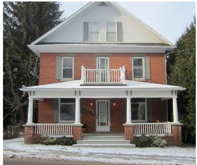
Existing residential dwelling that illustrates entry elements such as porches and generous overhangs to articulate front elevations at entrances.
