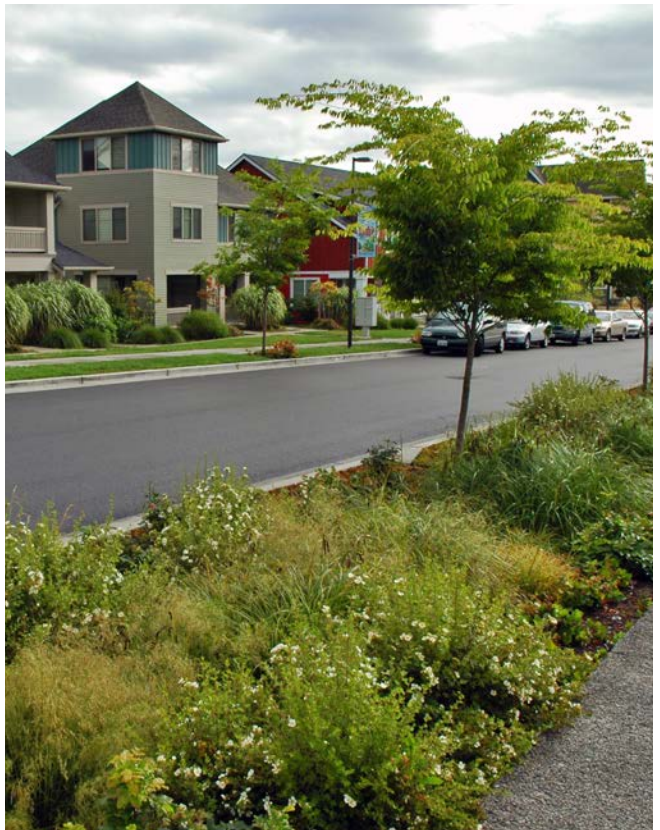
Local Road with a bioswale in the right-of-way to assist with run-off and infiltration.
