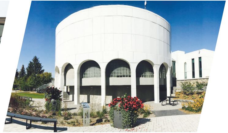
Civic Centre Accessibility & Green Courtyard Parks & Recreation Ontario Award of Excellence Park and Facility Design
